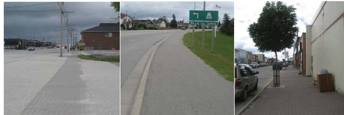
EXISTING SIDEWALK PAVING IN HEARST
