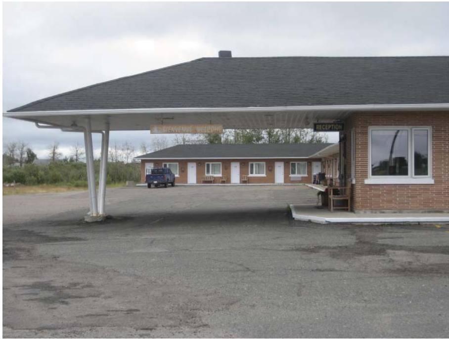
EXISTING - WELL-DEFINED ROOF LINE AND OVERHANG THAT PROTECTS AGAINST THE ELEMENTS
