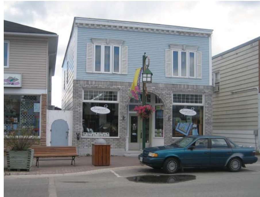
EXISTING - WELL-DEFINED ROOF LINE WITH CORNICE; PRIVACY DISTINCTION FOR SECOND FLOOR WITH MATERIAL CHANGE; WELL-PROPORTIONED WINDOW OPENINGS
