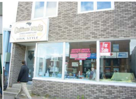
GOOD SHOPFRONT AND ENTRANCE; OUT OF PROPORTION SIGN
