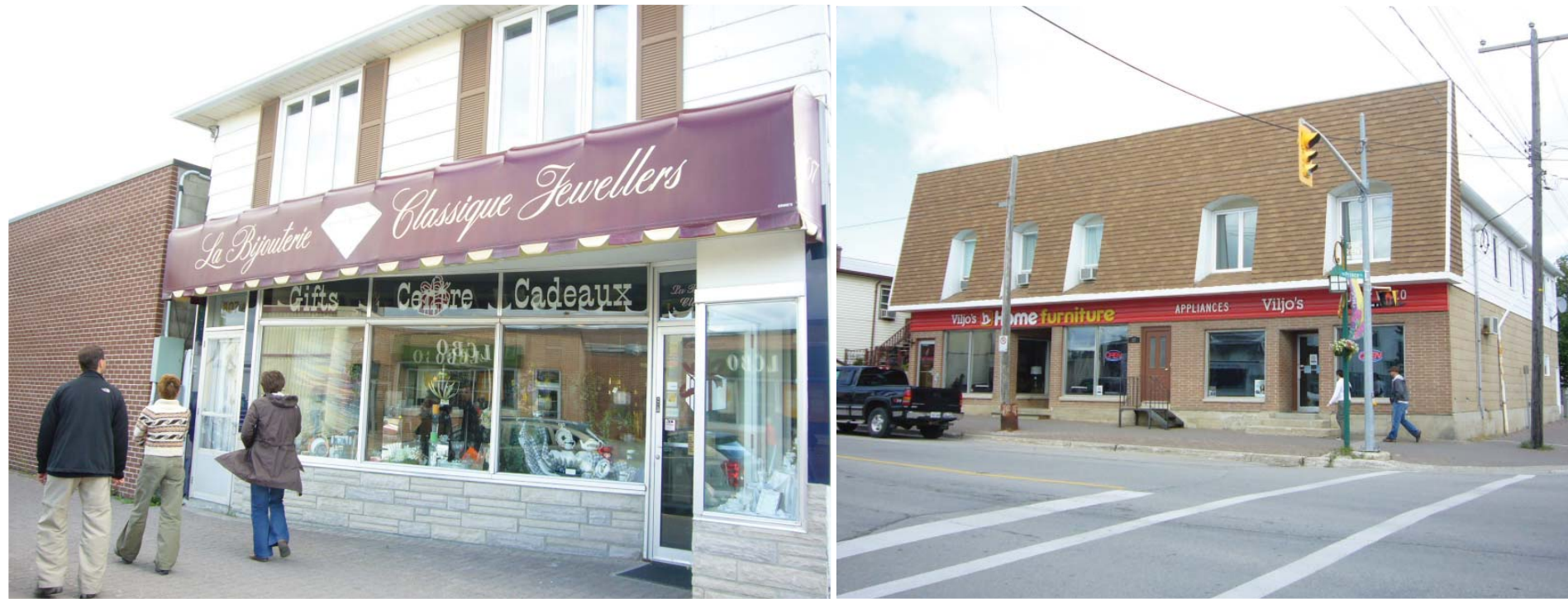
EXISTING CONDITIONS - EXAMPLES OF GOOD FAÇADES
